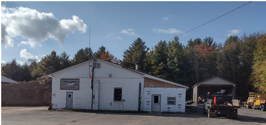
Town Highway Garage
