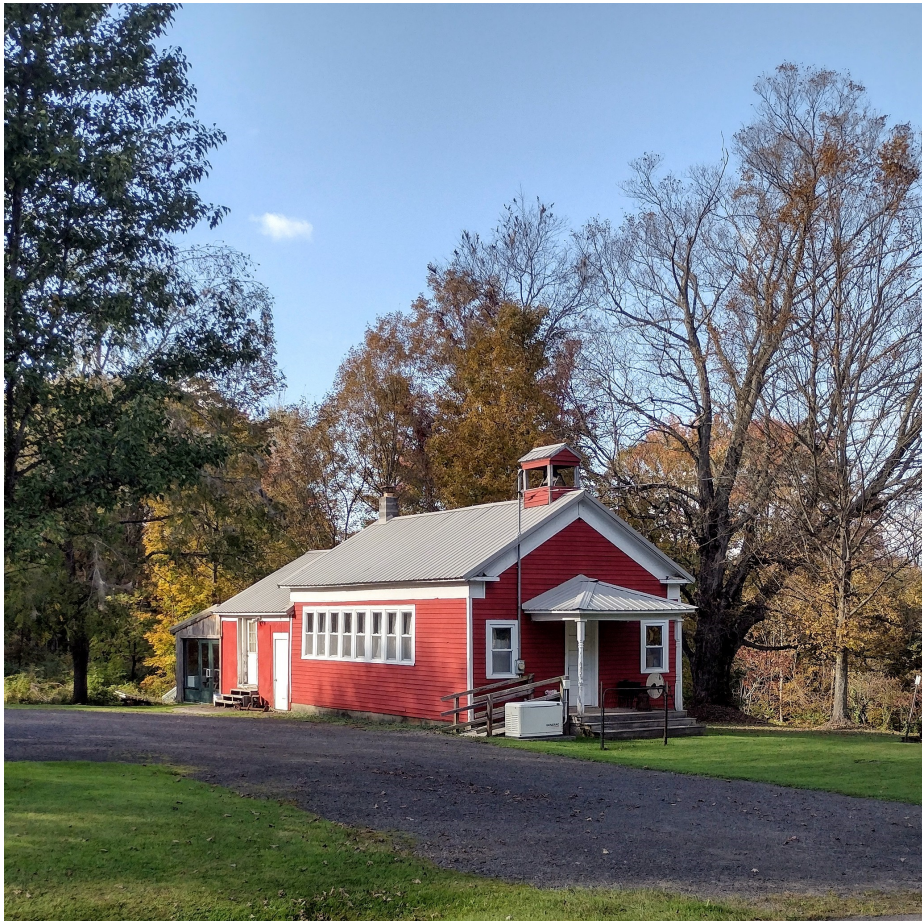
Amboy District No. 2 Schoolhouse
