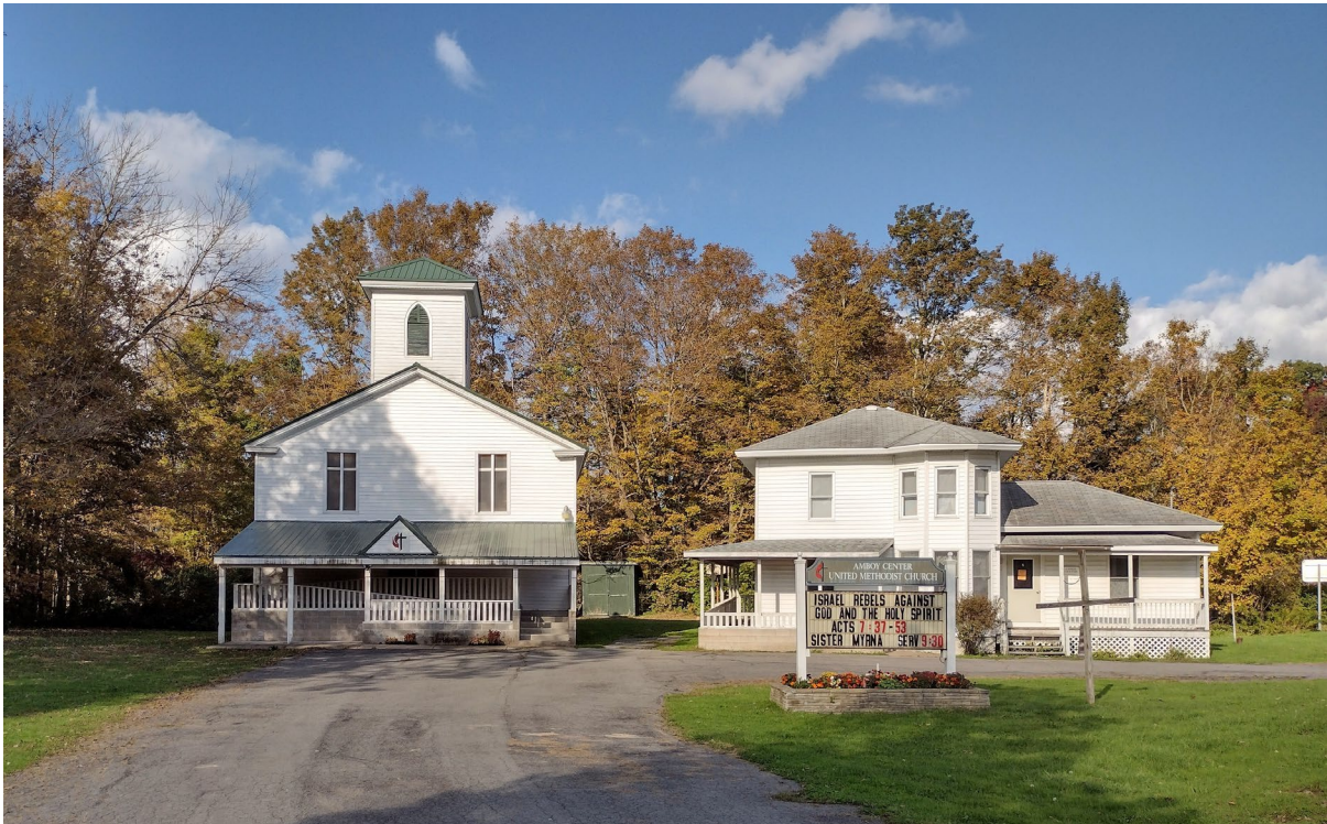
Amboy Center United Methodist Church
